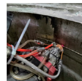
Bottom ring on-site repair
