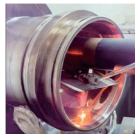
Cylinder liner repair
