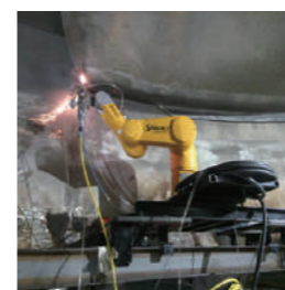
Hydro-power turbine coating
