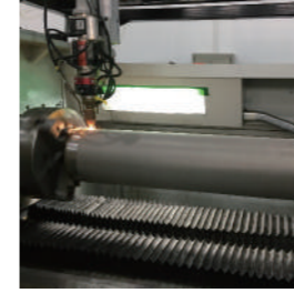
Hydraulic support column repair
